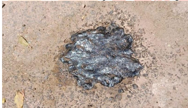
Fig. 10. Filling of pothole with our product
