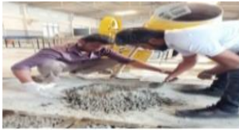
Fig 8. Mixing of materials
