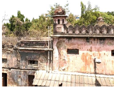
Figure 2 Condition of the façade.
