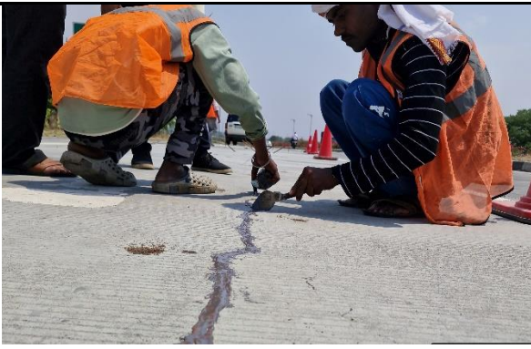
Fig. 3. Sealing of the cracks with Polysulphide base sealants
