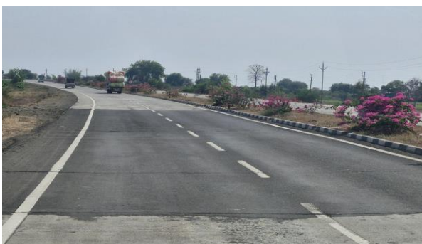
Fig. 4. Over Laying of Bitmine Concrte layer on the PQC
