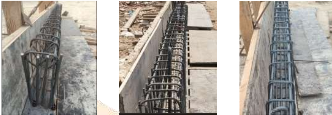
Fig. 2 Configuration of two-piece, U-shaped, and closed stirrup on site.
