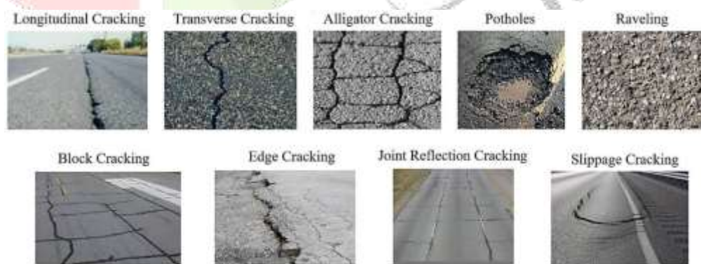
Figure 1: Multiple types of road pavement failures [12].
