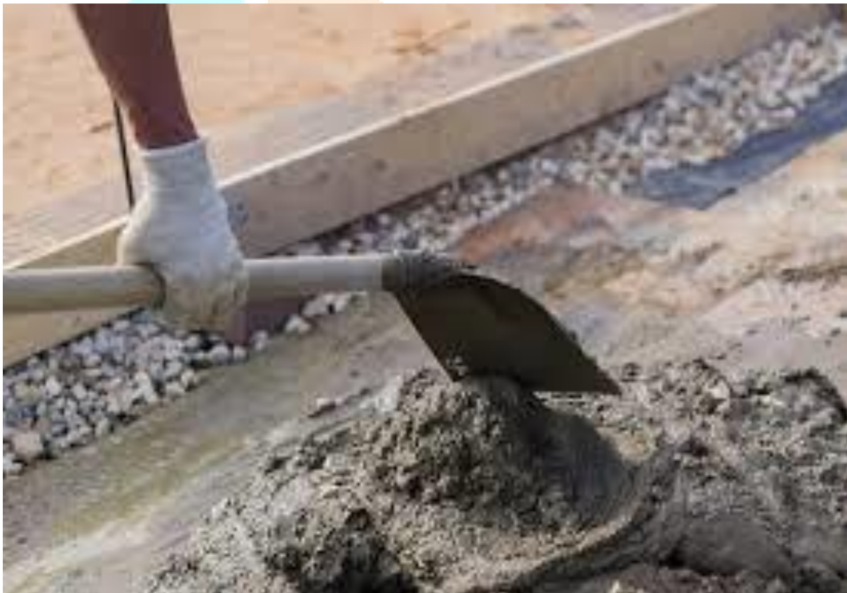
Figure 3.1: Mixing of Concrete
