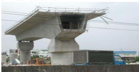
Figure1.1 Box Girder Bridge
