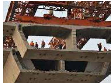
Figure. 1.2 Double Cell – Box Girder
