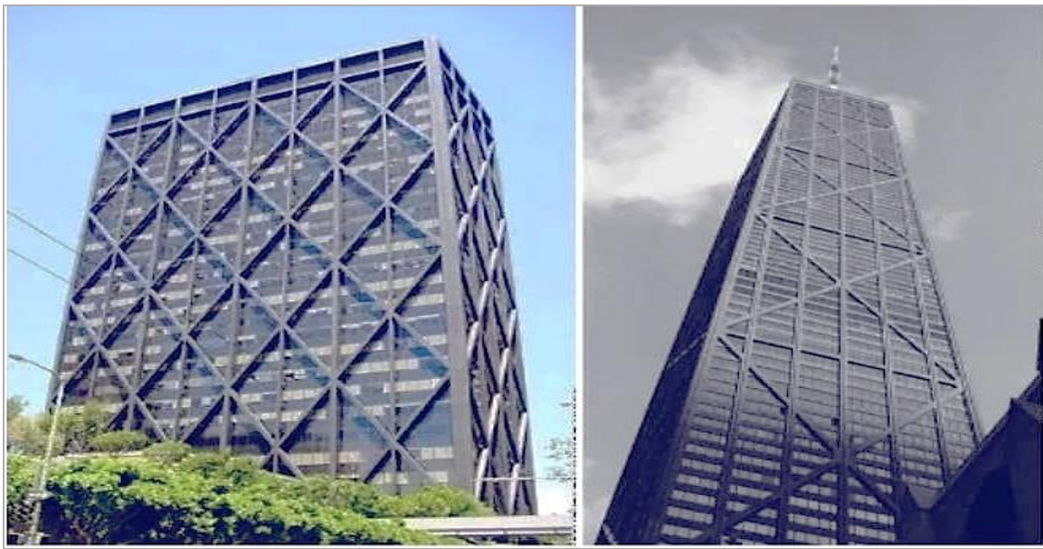
Figure 2 braced frame structure
