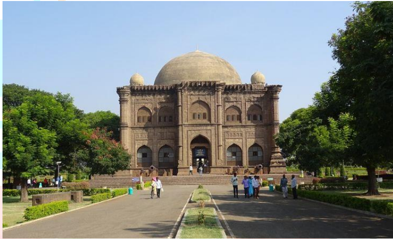
Fig 2: The surrounding gardens, entrance gateway and enclosure of Gol Gumbaz complex.
