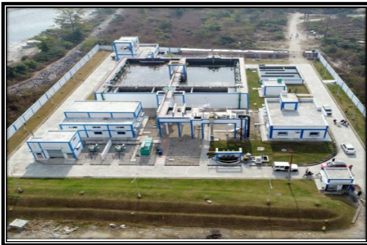
Fig.1; Sewage treatment plant (STPs) is located at Ramnagar, Nainital
