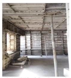
Fig No. 1 Aluminium Formwork
