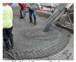
Fig No. 4 Concrete Pouring
