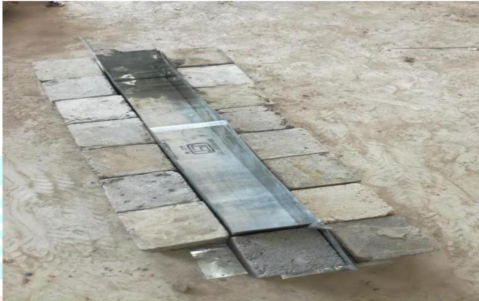
Figure 7.1 : RC Beam mould preparation
