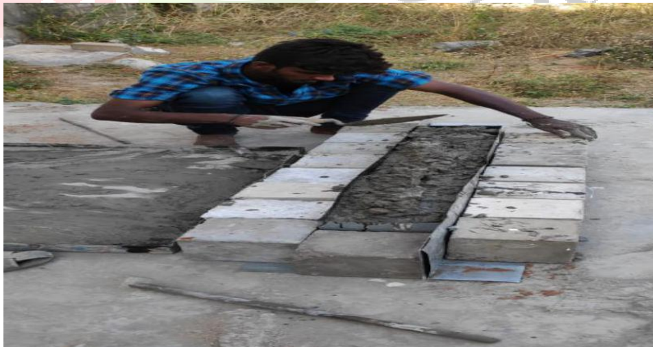
Figure 7.2 : Casting of RC Beams
