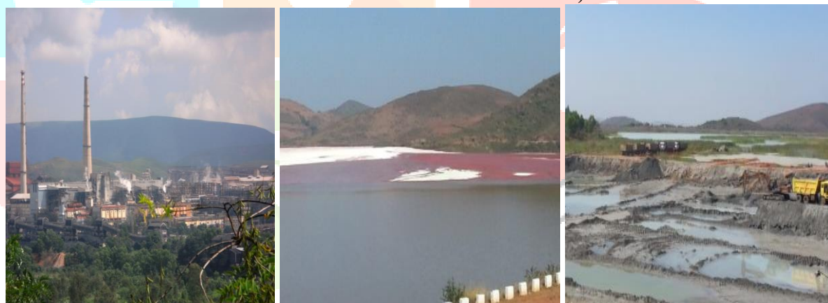
(Photographs: NALCO industry, Red mud pond and lechate leaking from the dam site)
