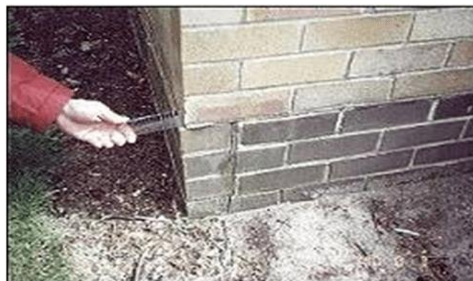
Fig 1: Effect of sulphate attack
