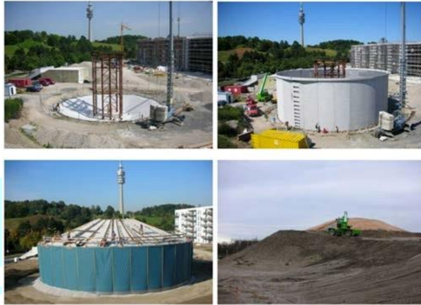
Figure 2 Construction of a tank thermal energy storage system in Munich, Germany [17]
