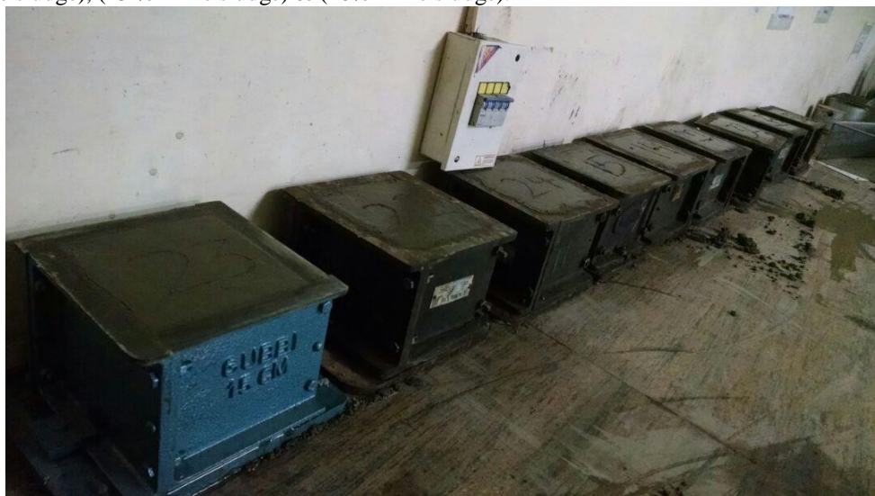
Figure 4.1: Casting concrete blocks in moulds
