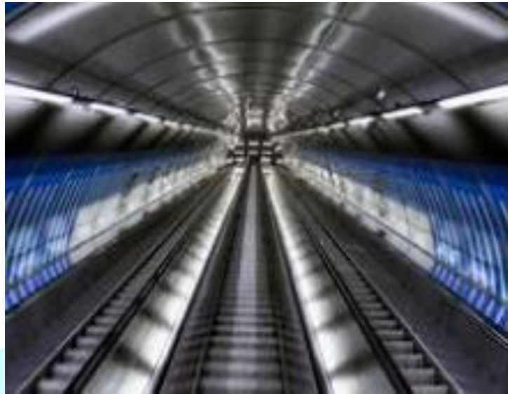
Fig. 5: The tunnel for the Barcelona Metro Line 9
