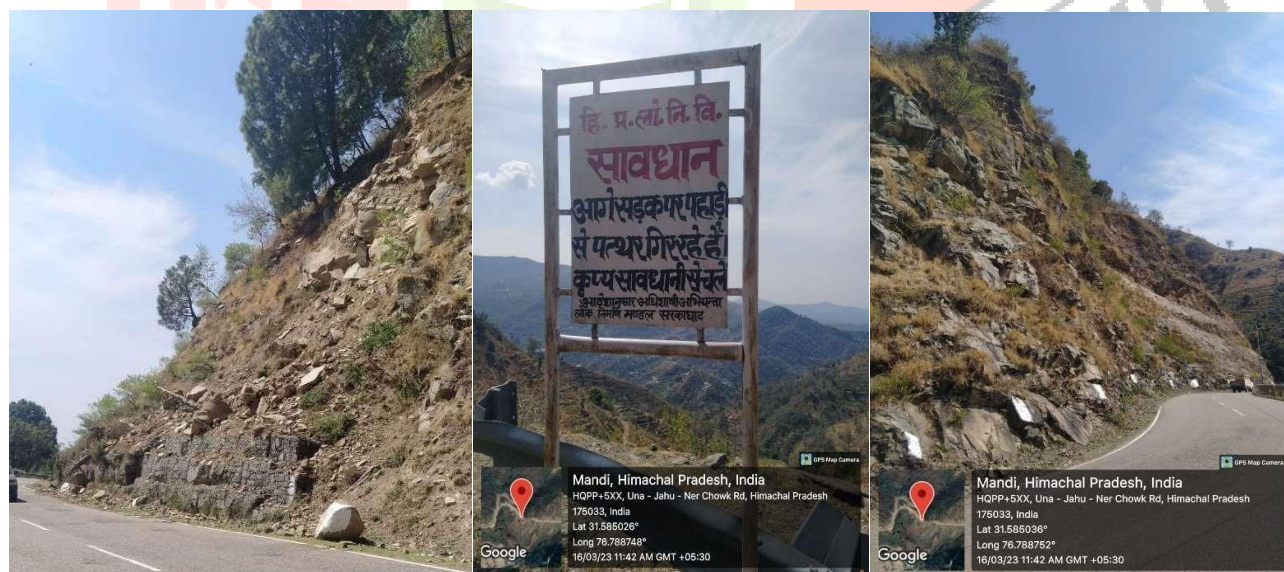
Figure 17: Some Photo of Rock falling Zones
