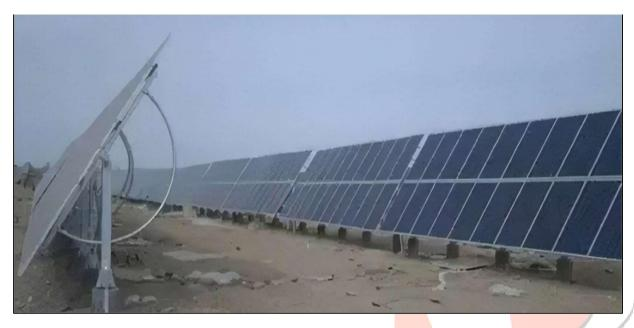
Figure 2. Tilt angle Adjustment for More power generation
