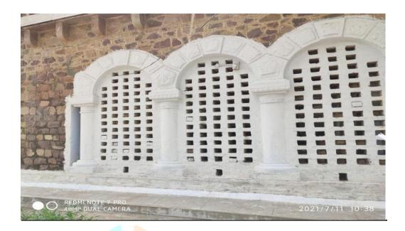
The church building comprises three pairs of reticulated Arch shaped windows running parallel to each other in a North-South direction. The main purpose of such direction is to provide proper ventilation by allowing healthy air from the height of the window, which is 7'10" and breadth, which is 4'5".
