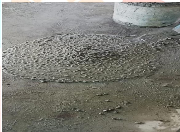
Fig. F. 1 Slump Flow Testing
