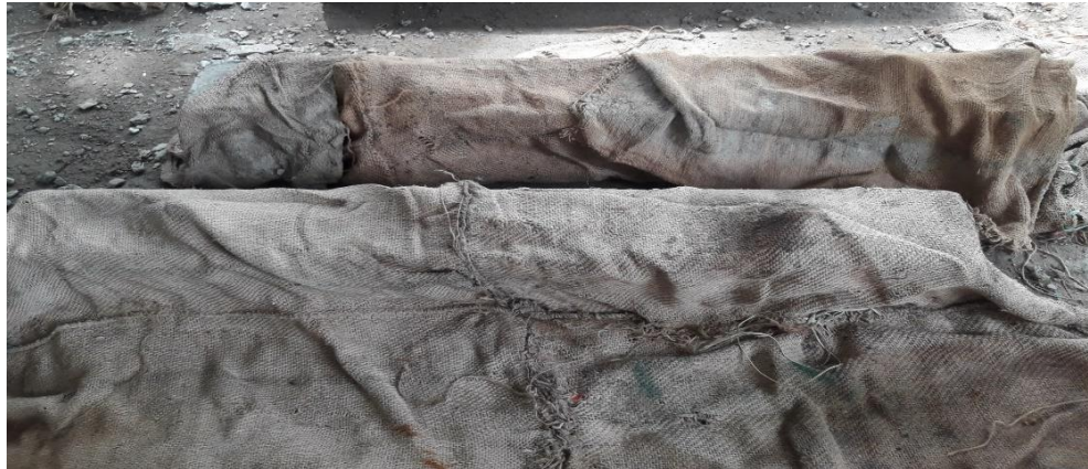
Fig. 5.4 Curing of Beams
