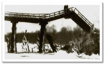
Buckling of bridge due to compression induced by earthquake
