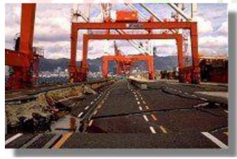
Lateral displacement of a quay wall, Kobe 1995
