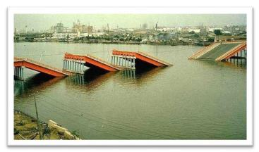
Loss of support due to sliding of soil during earthquake
