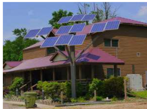
Figure 5 Mounting of Solar Tree near the house
