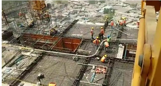
Fig no 4.1: tunnel form construction at central revenue quarters, Anna nagar west, Chennai
