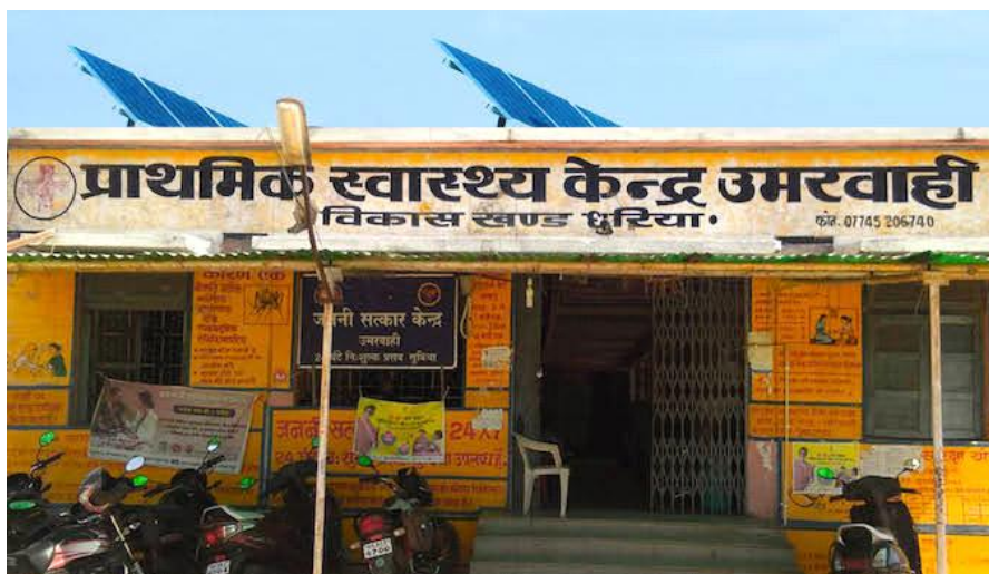
Fig 3. Fully solarised PHC in Chhattisgarh
