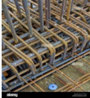
Fig 4. Congested Reinforcement in Raft
