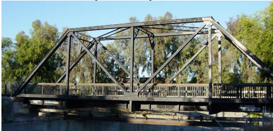
Fig. 1: skeleton of a typical steel truss bridge
