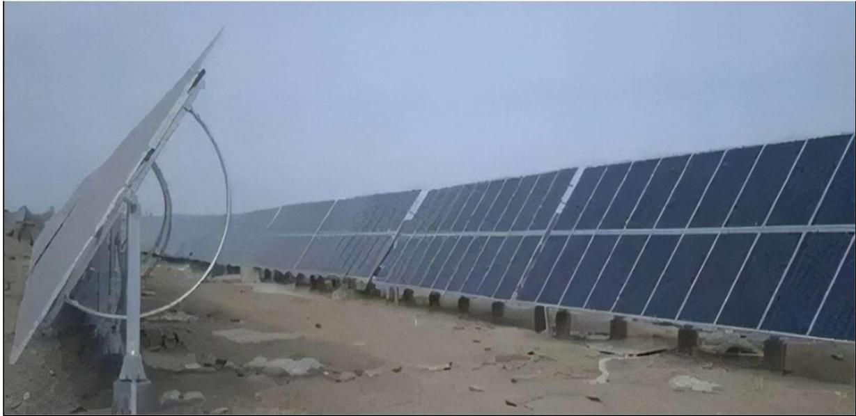
Figure 2. Tilt angle Adjustment for More power generation
