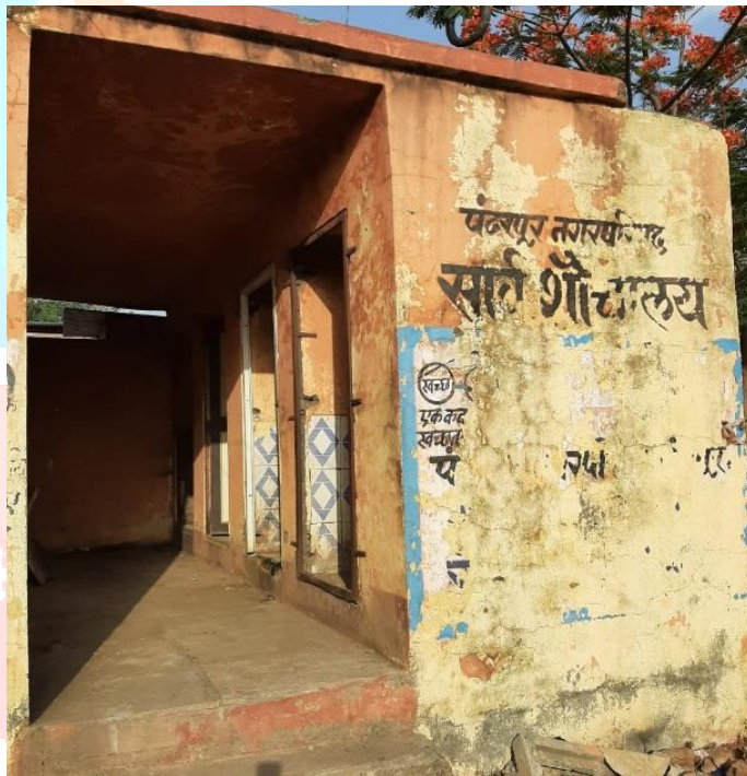
Figure 2 Exterior of public toilet (Source: primary source)
