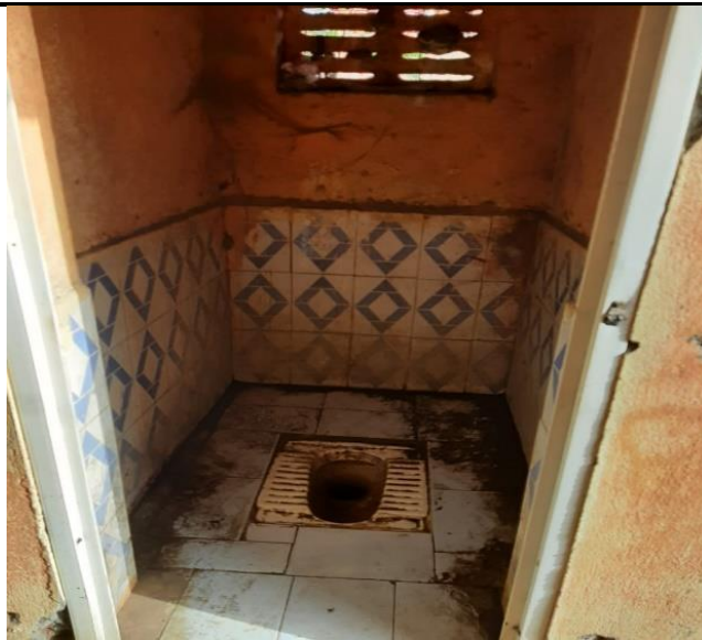
Figure 1 Interior of existing toilets (Source: primary source)
