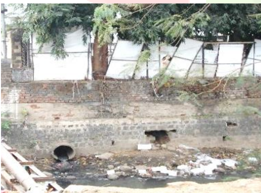
Photograph-5: Photograph of Wastewater discharge point at VIP road, Nagpur
