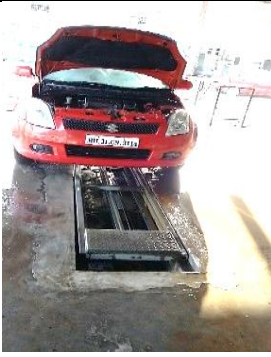
Photograph-1: Ramp with underground tank for wastewater collection at Seva Automotive, Nagpur.
