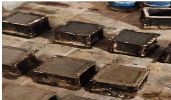
Fig: Casting of Concrete Blocks
