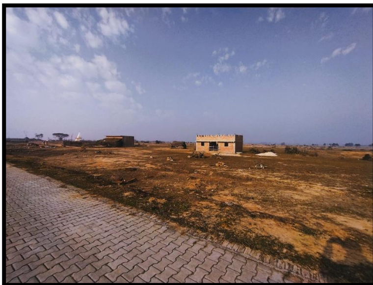
construction work just in front of main gate of sanctuary
