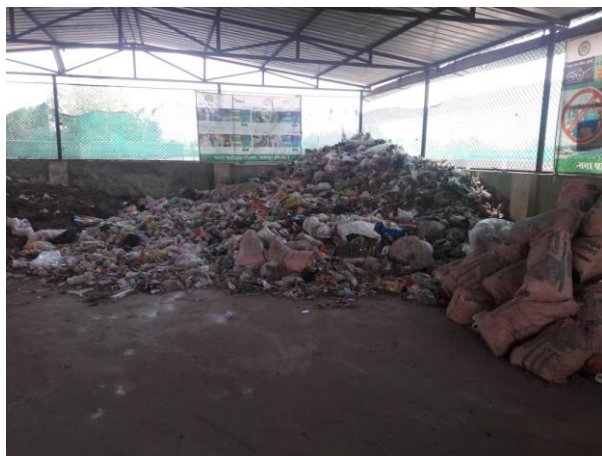
Transfer station – Devpuri, Raipur.
