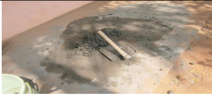
Fig.8.1 shows the hand mixing of concrete
