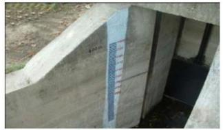
Figure-15 Water Level Gauge
