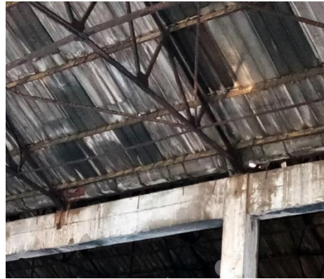
Existing Roof Truss
