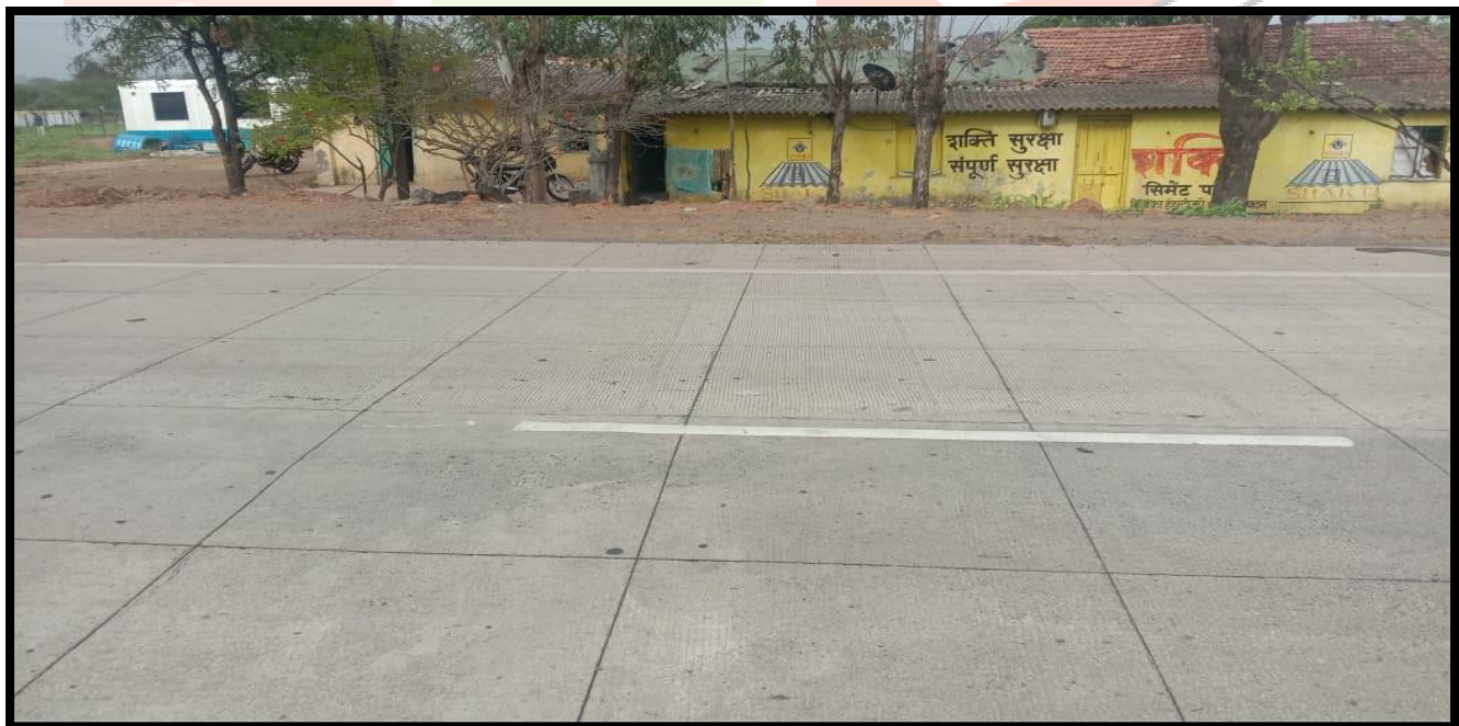
Figure 4.1: white topping road after finishing
