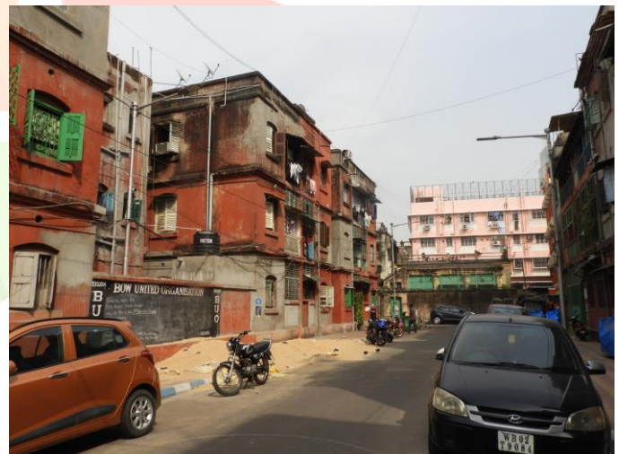
plastering over damaged surface
