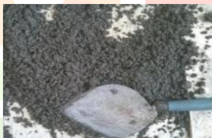
Fig 3 Mixing of dry ingredients
