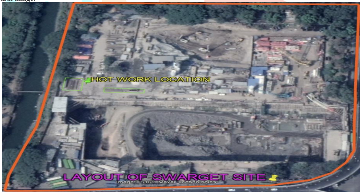
(Photo 01: Hot work Location in layout of swargate underground metro station pune)
