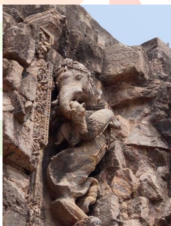
Figure 5 Fitted Sculpture by Consolidation Method
