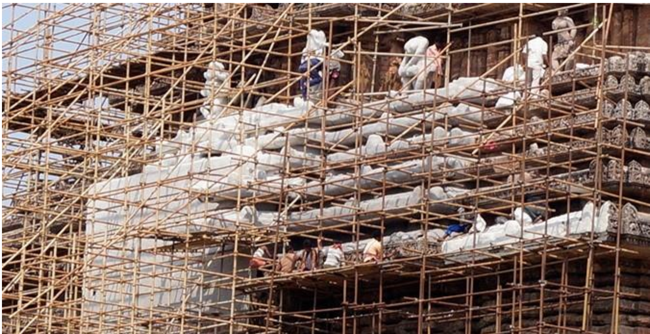
Figure 3 Desalination work under progress with Paper Poultice Method
