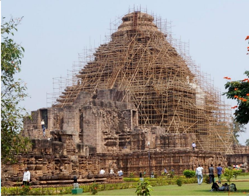
Figure 1 General view of the Pida Deul of the Sun Temple Konark
