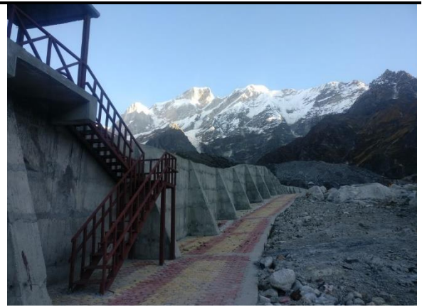
Fig 15. Retaining wall along Mandakaini River
