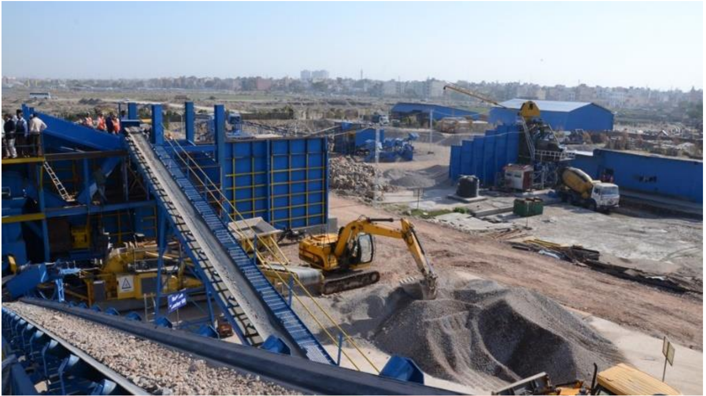
Fig 5. Burari Recycle Plant
