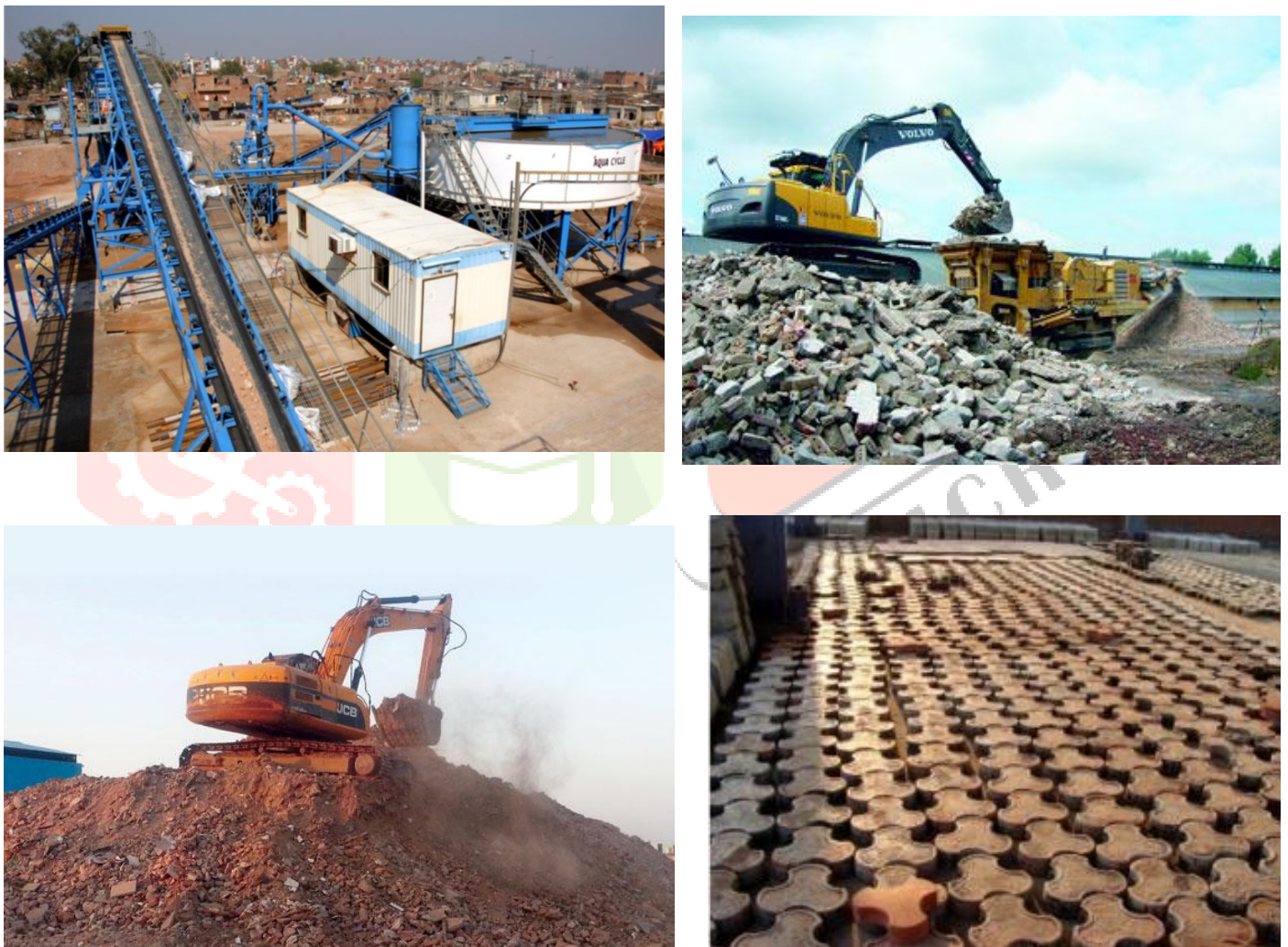
Fig 7: Photographs of Construction & Demolition waste processing facility at Burari, Delhi
