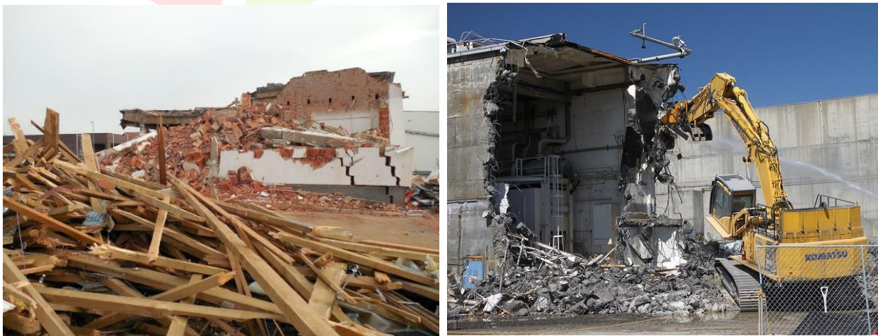
Fig 1. Debris generated from demolition
