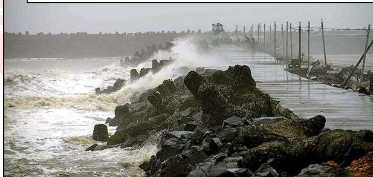
Breaking of the boulders due to excessive swash of the tides and flooding of the roads
