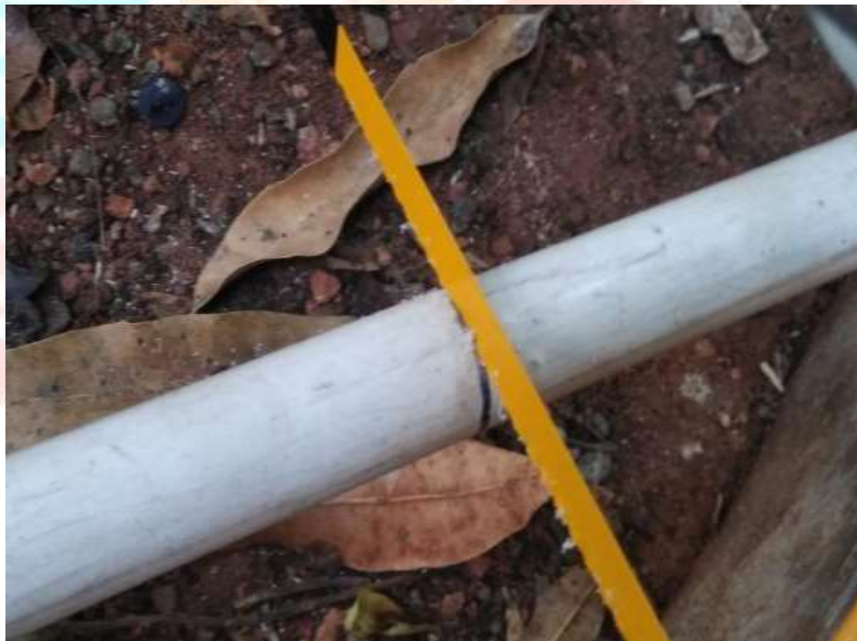
Fig -4: Cutting of UPVC Tubes
