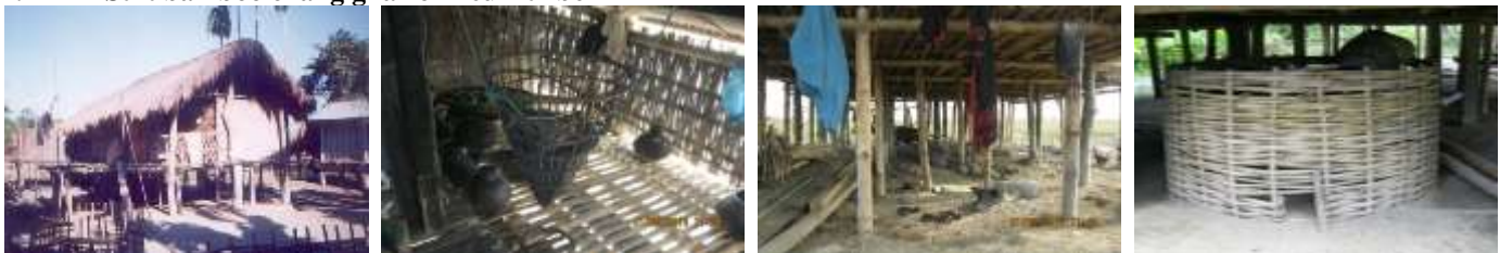
Fig : 24 Deuri chang ghar, perforated floor, pig stay and duckery under the stilt
