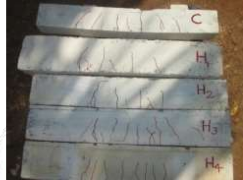
Fig.4 Failure mode of specimen
