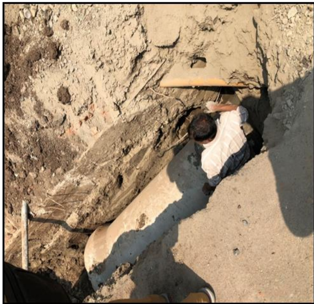
Fig no 5:- RCC laying work
