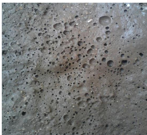
Fig 4 Surface preparation of Foam Concrete
